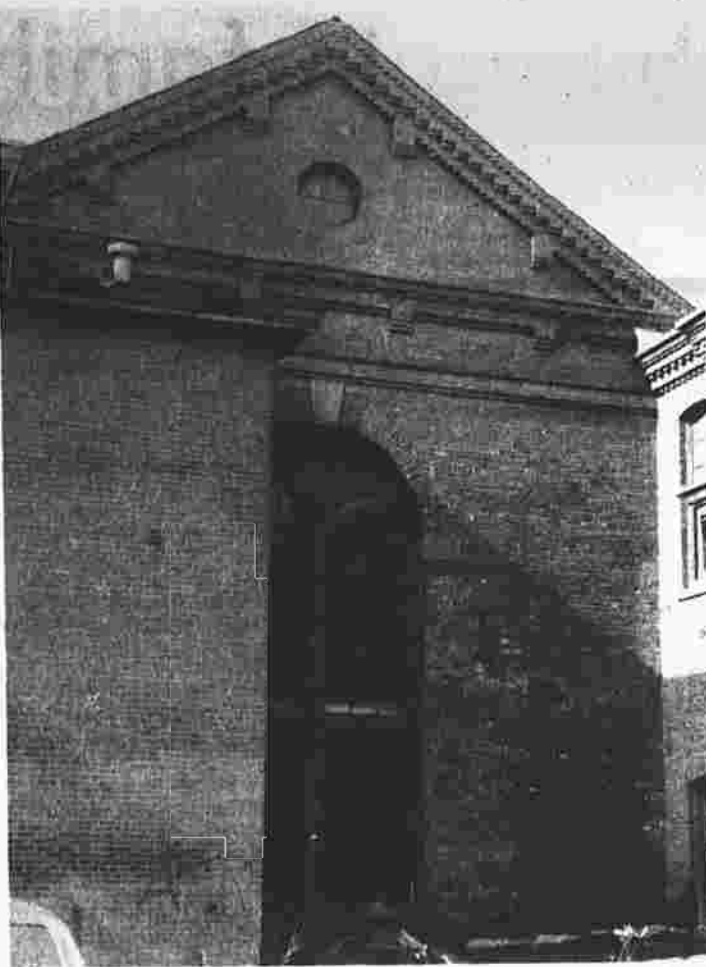
A view of the old chapel from the outside, shows that the structure was probably sandwiched between two mill buildings sometime after they were built.
